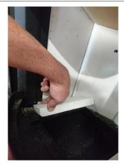
Remove grate and base fire bricks.
