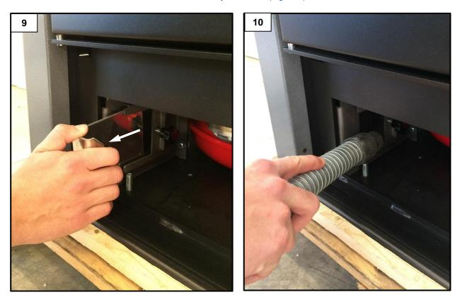
After unscrewing the hand-wheels, extract the side flue gas pass inspection vent (Figure 9). Remove the deposits inside using a suitable ash vacuum device (Figure 10). When finished, close the pipes making sure that you have secured the two inspection openings. Replace the front panel below.
