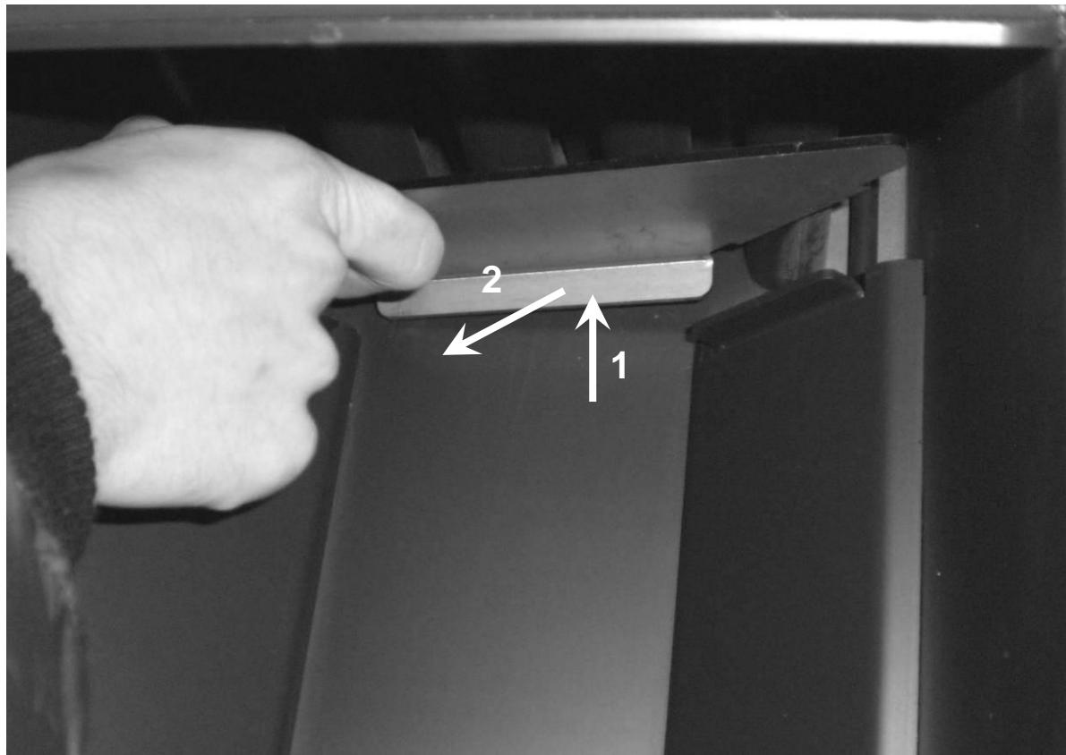
Remove the flue gas deflector located above the combustion chamber. Firstly, pull front knob to remove the deflector.
