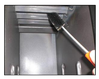
With the supplied brush clean the elements on the combustion chamber. These can be accessed through the combustion chamber.
