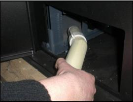
Open the hatch under the pellet side and, after having loosened the hand wheel, extract the plate from the lateral "flue gas pass".
