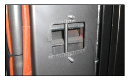
Clean any obstructions in the lateral fumes passage and re-mount the inspection outlet.
