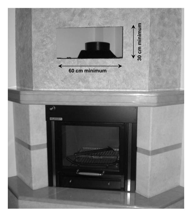
The inspection hole can be covered with a bracket or aeration grid.
