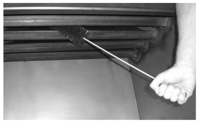
Use the brush supplied to clean the 4 slanted elements of the flue gas pass inside the combustion chamber.
